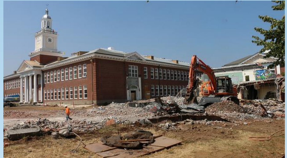
Phase 3 Work Underway at Old Cafeteria
