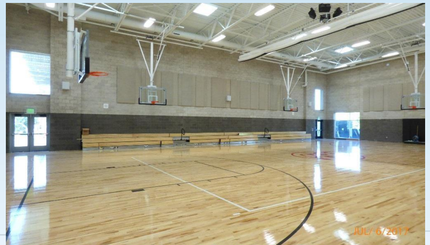
Gymnasium Bleachers Installed
